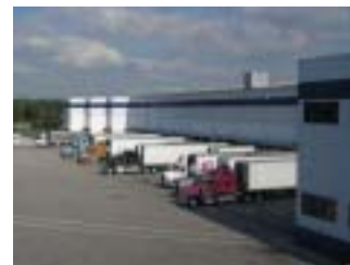
Sysco Loading Dock
